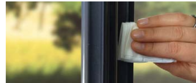
Maintenance of the gaskets
